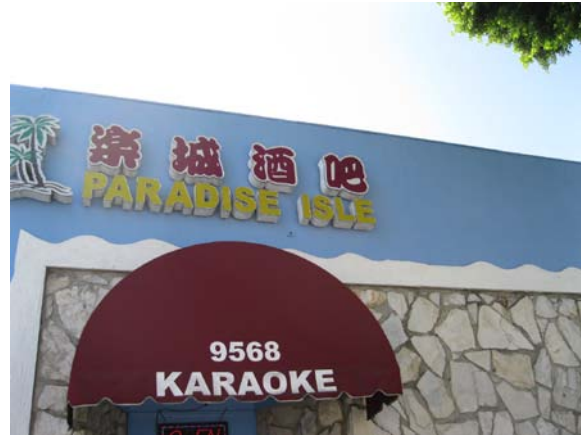
(After) Repainted front façade and repaired lighting.
