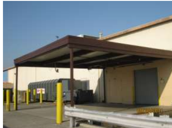
(After) Repainted patio cover.
