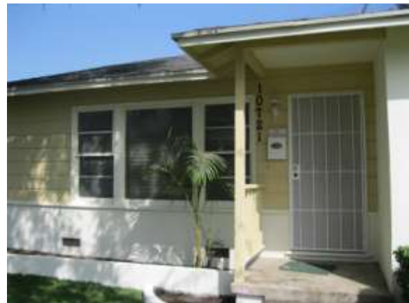
(After) Siding replaced, exterior repainted, and new door installed.
